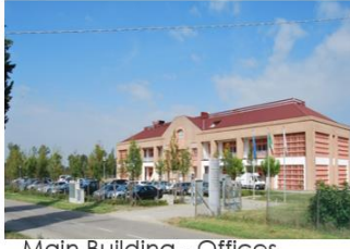
Main Building - Offices and Labs
